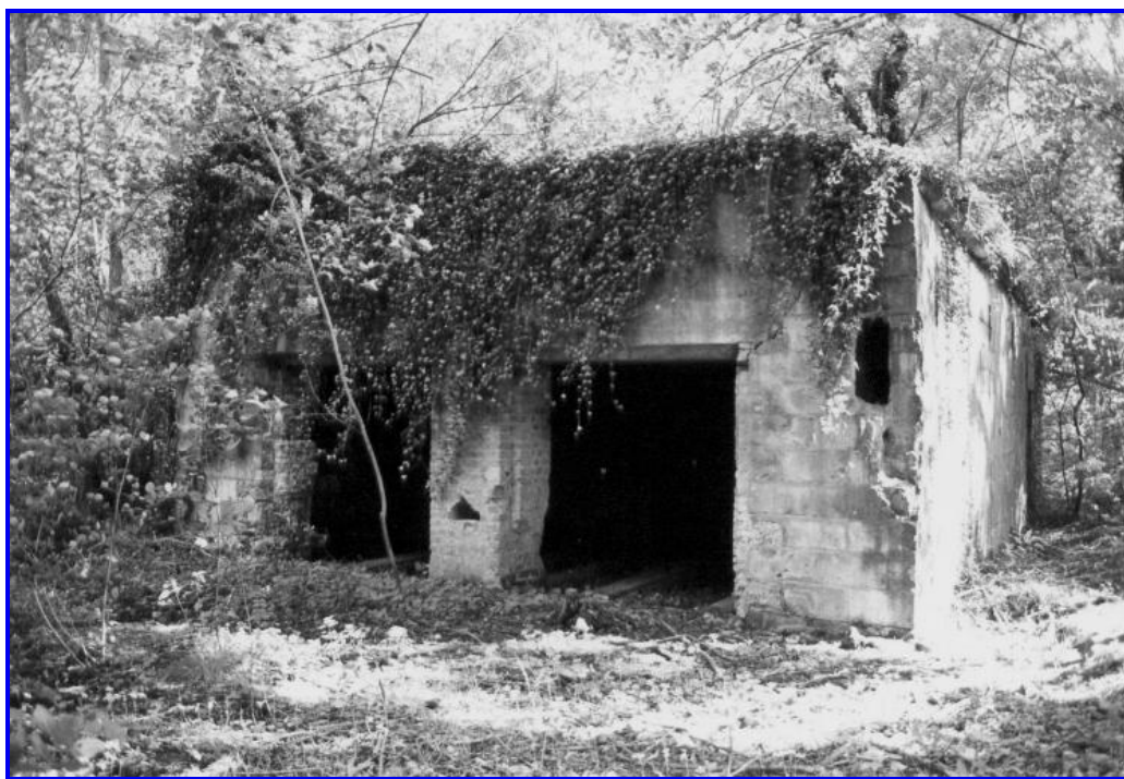
wpt 003: Compressor building: Place were the Dampferzuger was recycled and prepared for a new V1 Launch.
