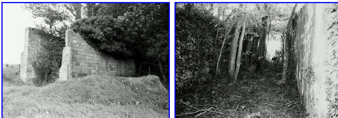
wpt 009: Launch Ramp with protective walls; front and backside. the front side is probably reduced in size although I am not sure of it.
