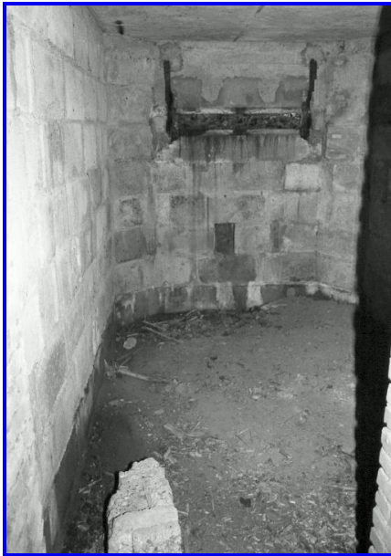
Fire Cabin wpt 008: In and outside.
